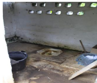
A toilet with brick walls and cement floor.
