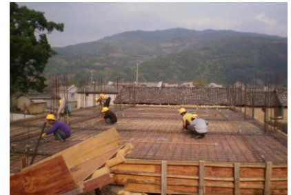
ChangAi team inspects school construction
